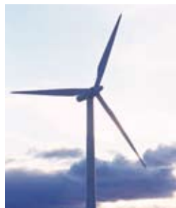
Large wind-power generation facility (reference photograph)
